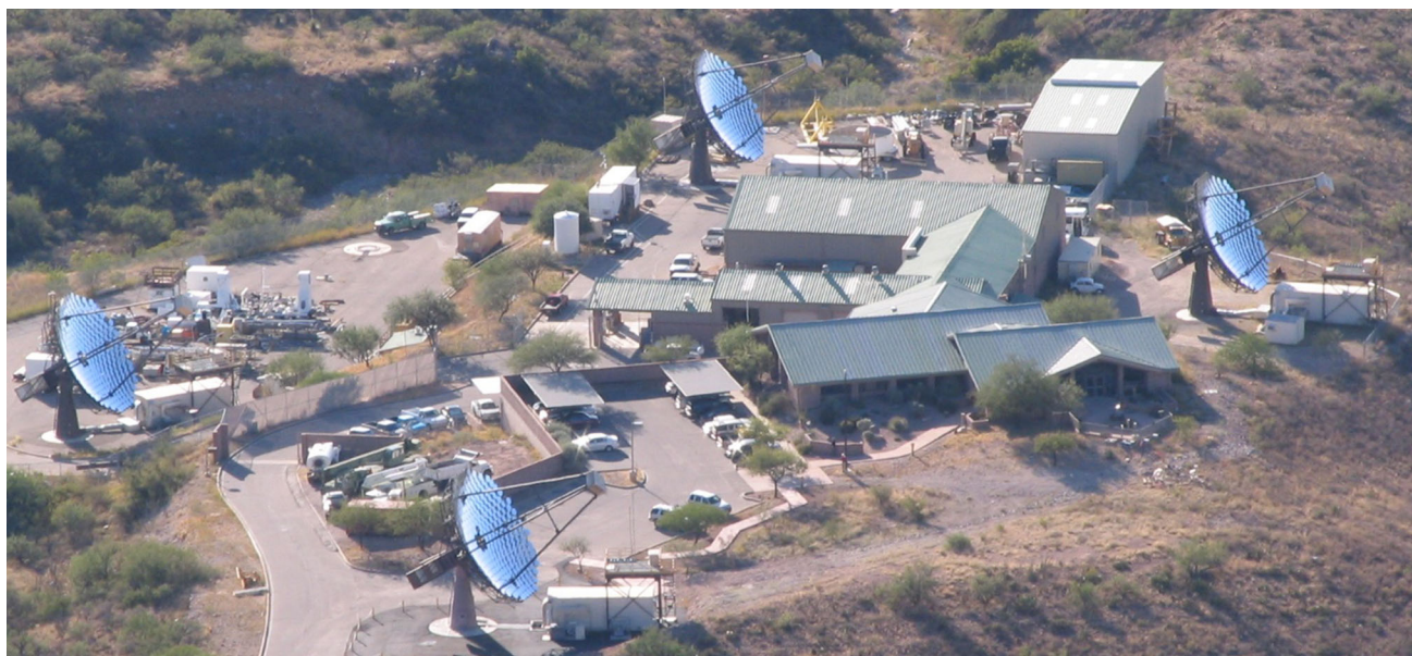
Fig. 12 VERITAS array in Arizona consisting of four 12-m-diameter telescopes. Picture courtesy: VERITAS collaboration
